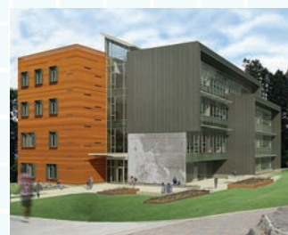
Construction is underway with Jabs Hall scheduled to open in fall 2015.
