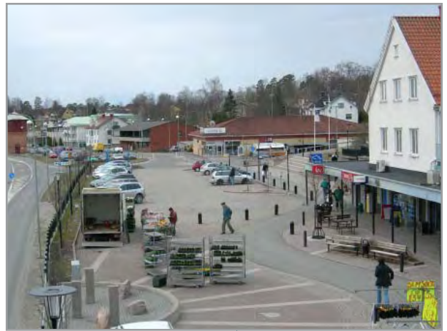
Opposite page: Mullsjø's modular pellet-fired district heating plant.
