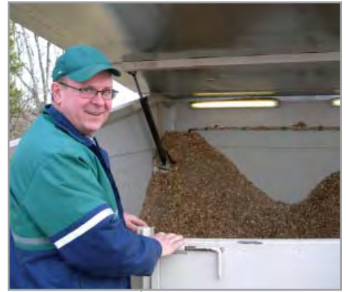
Opposite page: The small Koivulahti pre-fabricated Megakone central heating plant, the roof of which opens up to accept wood fuel deliveries.
