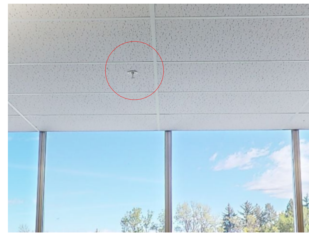
PHOTO OF EXISTING PENDANT SPRINKLERS ALONG NORTH WALL TO REMAIN, 5'-3" FROM GRID LINE A.
